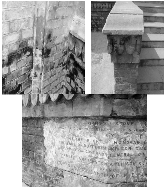
Figure 1.13: Seepages appeared on the brickwork on the entrance of the Old building of Aitchison College
