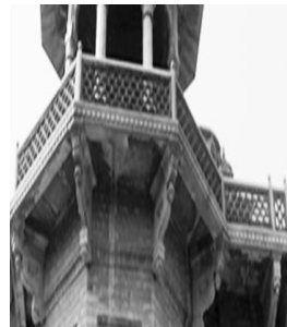
Figure 1.11 Redstone Jali of Parapet wall
