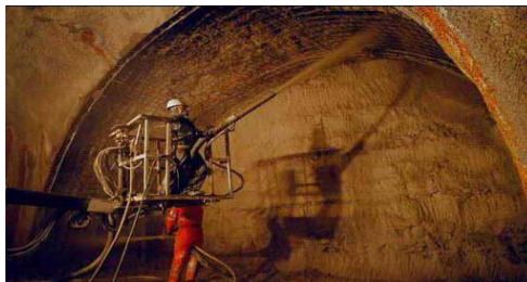
Fig.4. Applying layer of shotcrete
