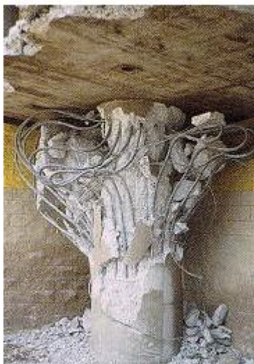
(Canyon Bridge Simi Valley San Fernand) Failure of column due to Buckling of main bars
