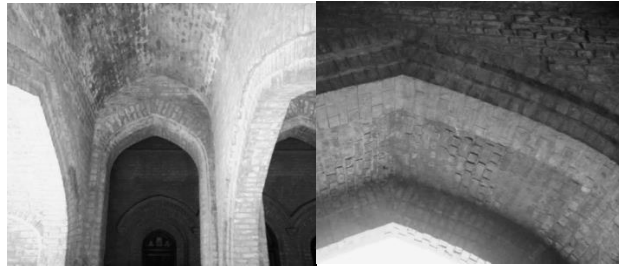
Figure 1.16: The efflorescence appeared on the ceiling of Aitchison College Old Building
