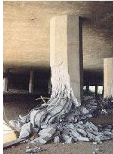
(Canyon Bridge Simi Valley San Fernand) Failure of column due to Buckling of main bars
