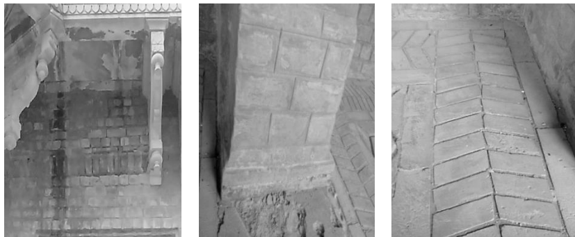
Figure 1.14: Deterioration of bricks has started due to dampness under the Balcony of Old Building and the hairline groves which cause the deterioration and efflorescence
