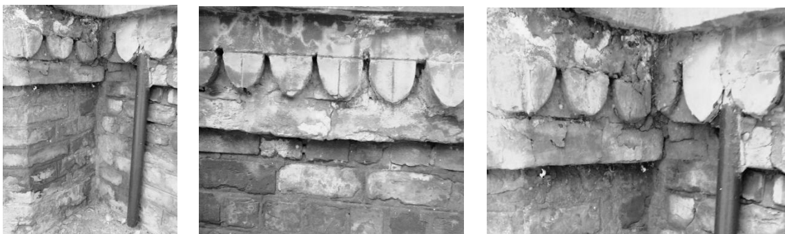
Figure 1.15: The efflorescence and deterioration appeared on the face of brickwork in the outer plinth of the Old building Aitchison College due to dampness
