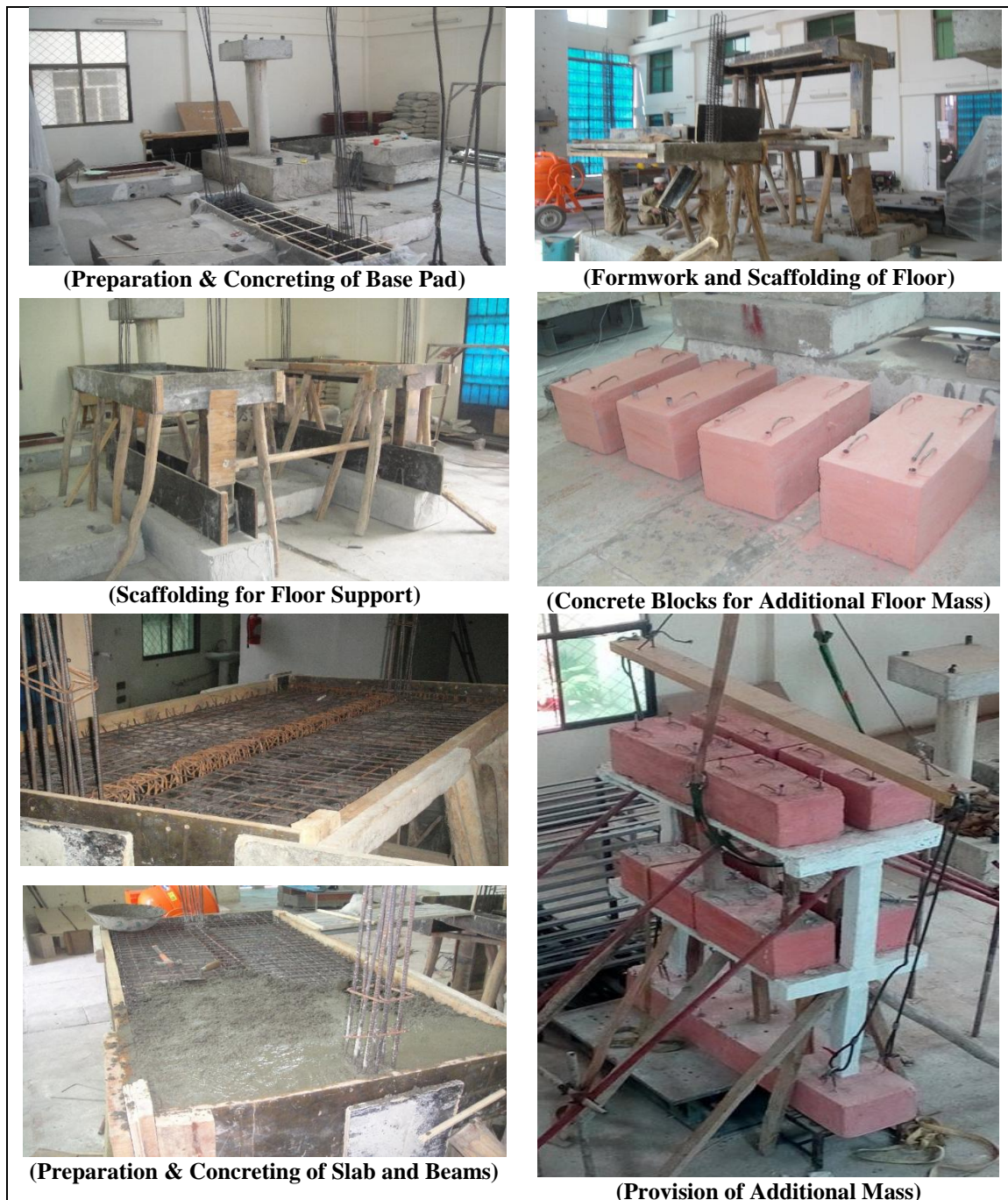
Figure 3: Construction Sequence of Test Model
