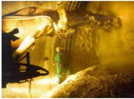
Fig.3. Cutting a length of tunnel with a road header
