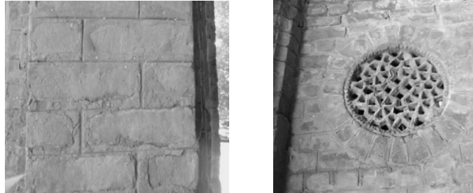
Figure 1.17: The deterioration of bricks in the column and on building facade of Aitchison College
