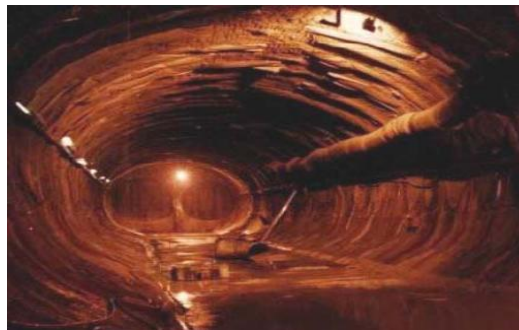
Fig.5 Primary lining applied to whole cavity which remains under observations
