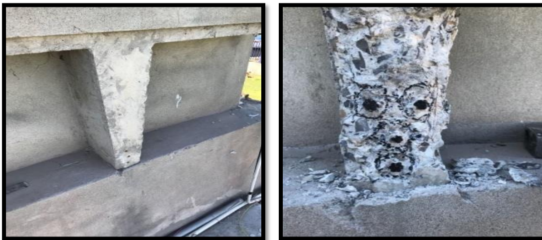
Figure 1 : (a) and (b) shows scratching of Tee Unit
